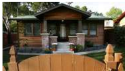
Remodeling a 1924 cottage in Eagle Rock
